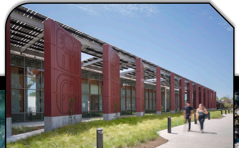
Sundt Construction – SWCCD Institutional Technology Building
